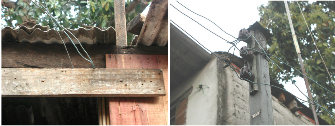
Figure 7: Unsafe energy connection pictured by the students
